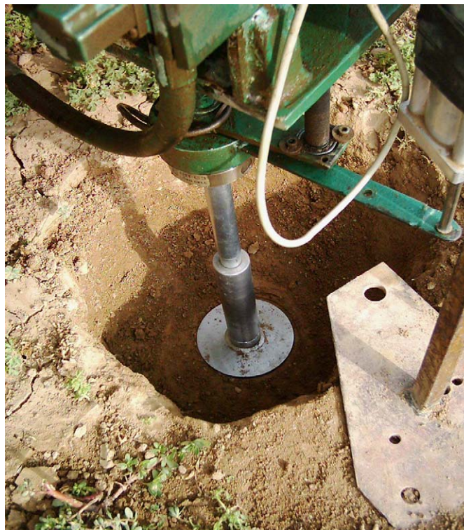
Fig. 3. Plate sinkage test on the subsoil
