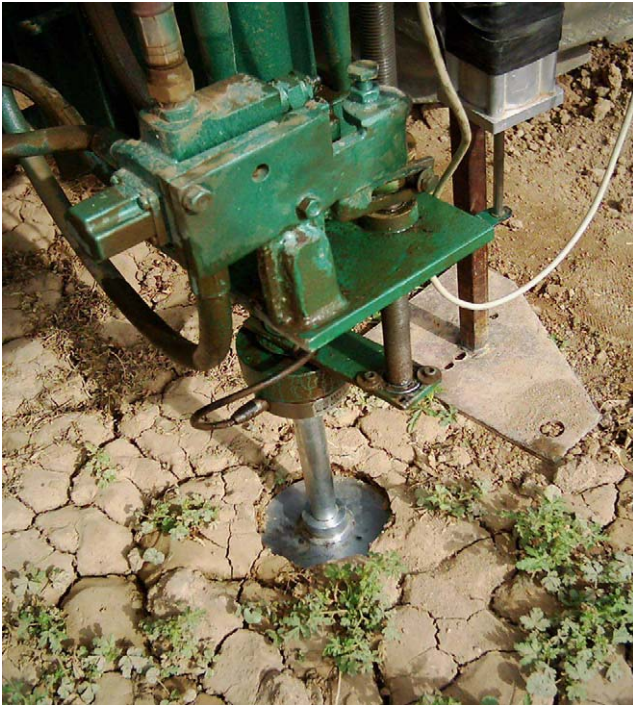
Fig. 2. Plate sinkage test on the topsoil
